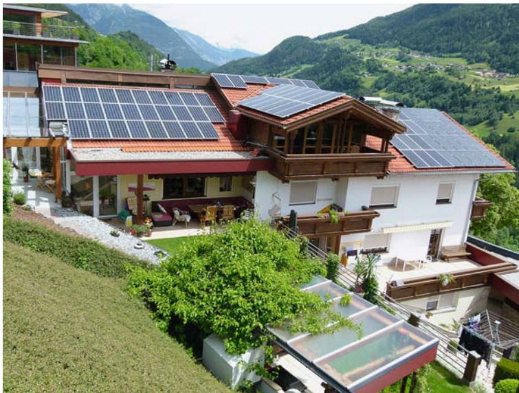
Picture 1: PV system on the building, source: Elektro Wultschnig
